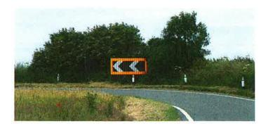
Road markings – these are in a worn condition. The double white line system for southbound traffic does not commence until the apex of the bend (photograph 2) allowing drivers the opportunity to overtake without an appropriate view ahead. The 'catseyes' within the white line system are in a poor condition and ineffective.
