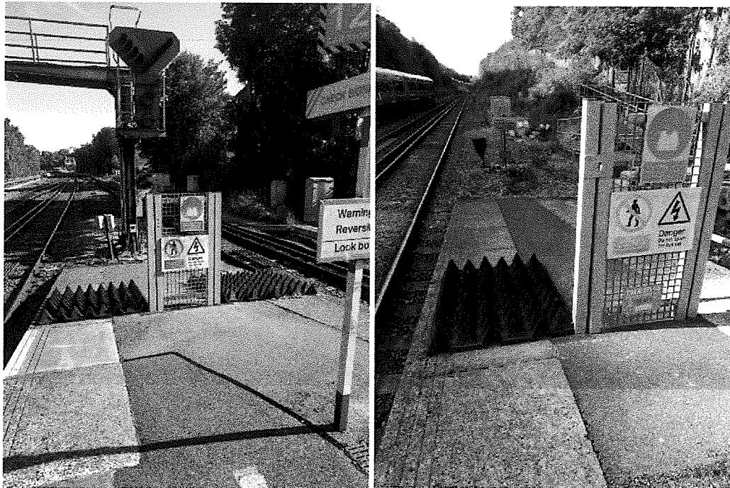
Preston Park Station
