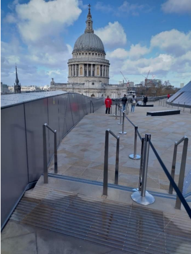
Image showing the two metre exclusion zone. 1
