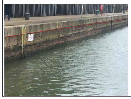
Railings are fixed at key points along the dock where there are corridors of open space, corners and intersections running perpendicular to the dock edge.
