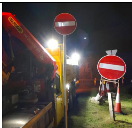
Image 2 - nearside sign rotated to the correct position on 26/04/2024
