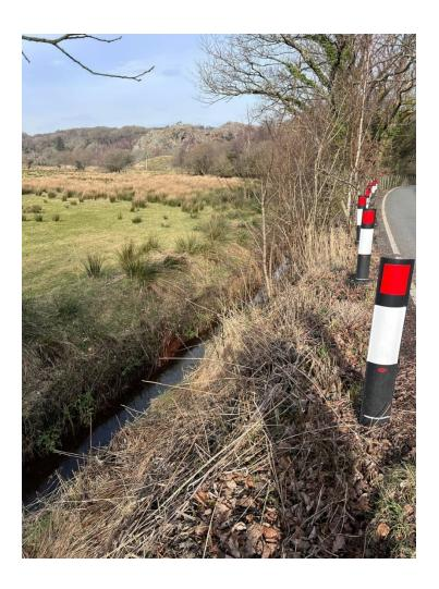
3.6 The bollards, whilst delineating the edge of the carriageway, are of low quality and unlikely to be sufficiently strong to prevent a vehicle crashing through them and potentially ending up in the ditch below.
