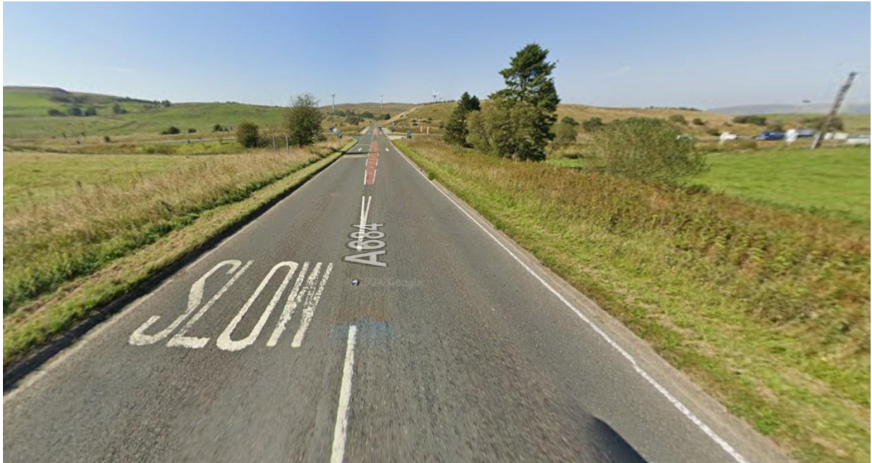
Prior to improvements A684 (Sept 2024)
